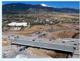
secondary span. The process maximizes the length of the bridge span and eliminates the need for another pier, which would
